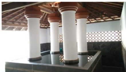
Figure 6. the four saka in the wudhu area
